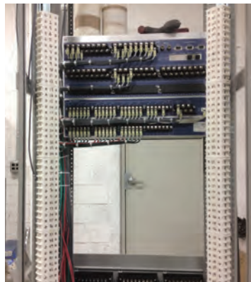
45° angled terminal blocks for ease of maintenance
